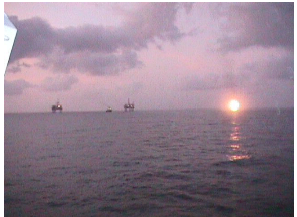
B-121 Gas Platform blow-out: 40 metre diameter fire-ball. Radiant heat felt at combat location 1 km distant.
