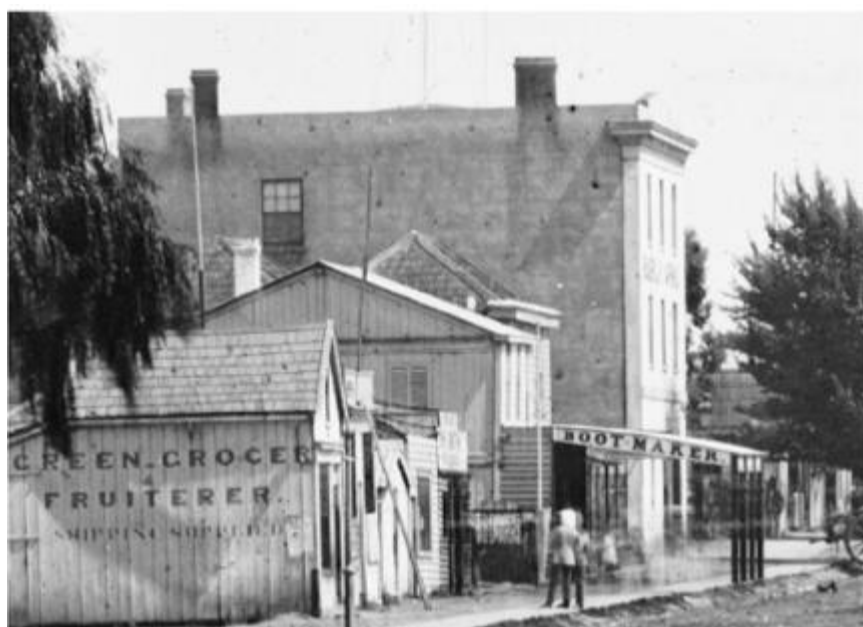
Detail of a view of Nelson Place, c1870-75, the former Oriental Hotel from the north-east, showing the heavy cornice and pediment that were removed in the early 20 th century (source: State Library of NSW)
