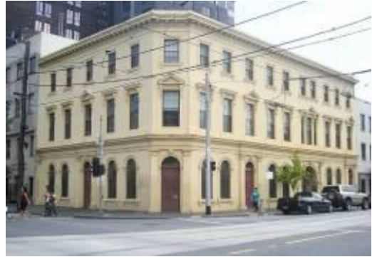
Former Eastern Hill Hotel, Fitzroy (VHR H0816) c1854-5
