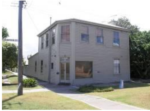
Bridge Hotel (VHR H1792), 1868
