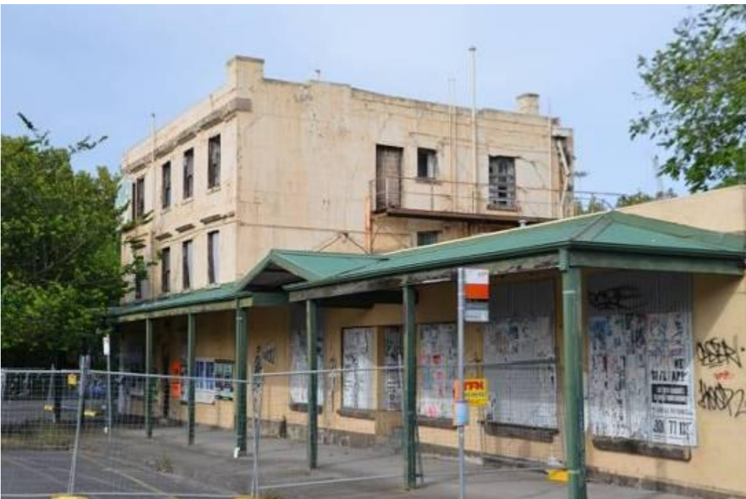
View of west elevation (Ann Street) from south-west
