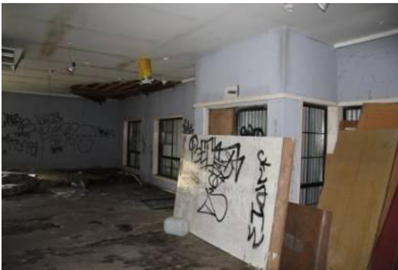
Views of the interior (source: Lovell Chen)
