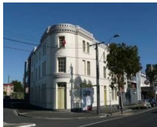
Former Terminus Hotel, Geelong (VHR H1162) 1853-54
