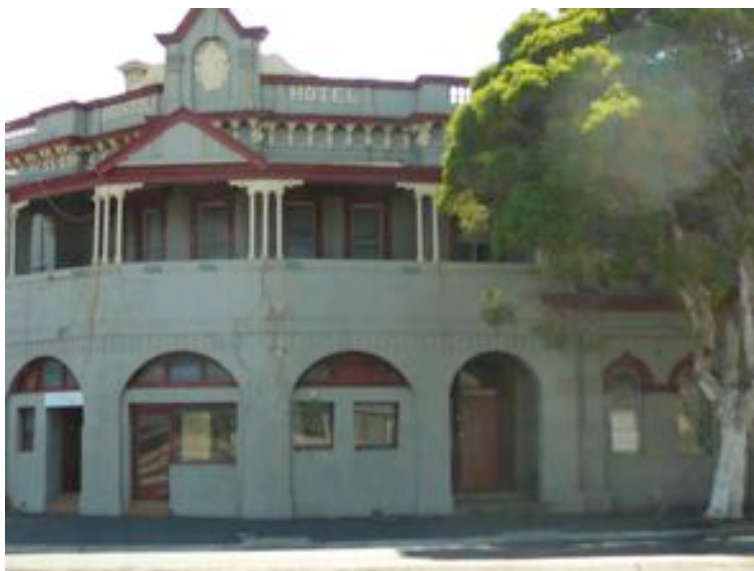
Figure 12. The Bristol Hotel in Ferguson Street. Note the extensive cracking and bulging to the façade.
