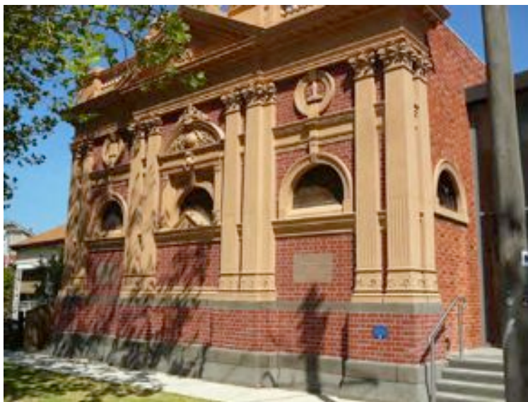
Figure 11. The recently repaired Masonic Lodge in Electra Street
