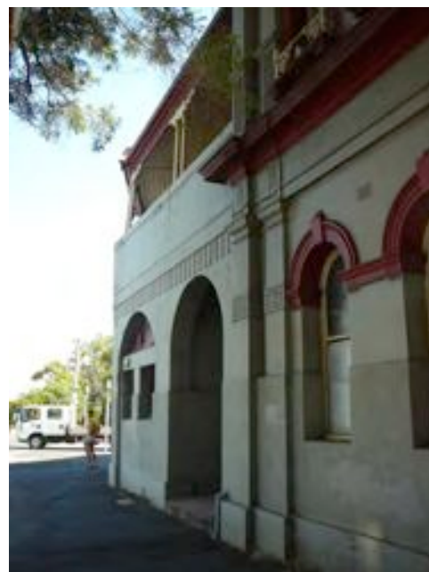
Figure 12. The Bristol Hotel in Ferguson Street. Note the extensive cracking and bulging to the façade.
