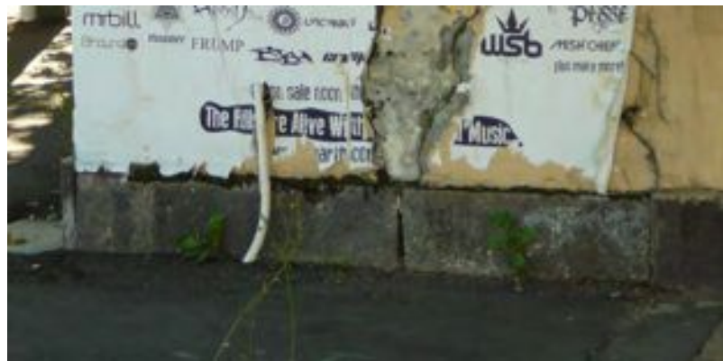
Figure 2. Bluestone blocks on Ann Street side
